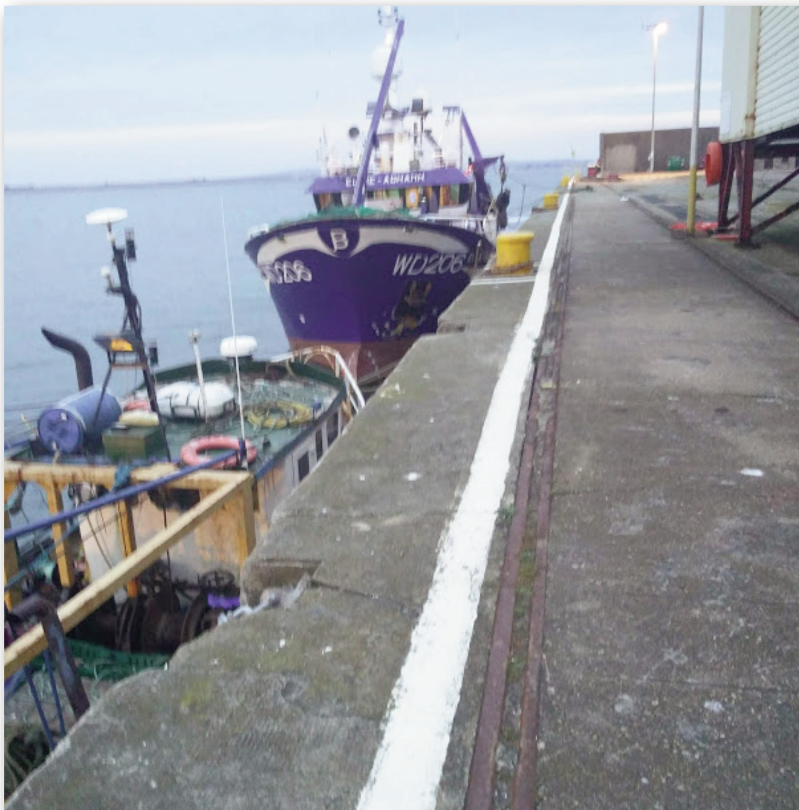
Photograph No. 4. No gangway or safety net were rigged and there is no clear designated access point between the 'MFV Ellie Adhamh' and the quay wall.
